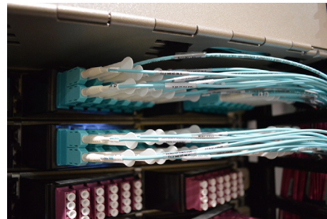
High-density patch cords that are easy to remove through the use of a flexible pull-tab
